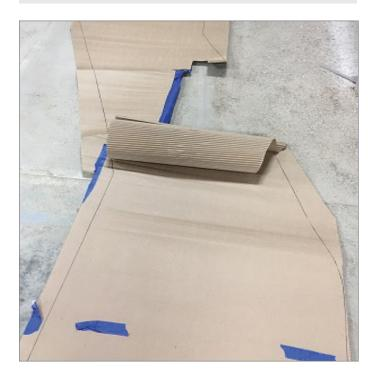
**Template material** — for best results countertop templates should be assembled using heavy corrugated cardboard.
